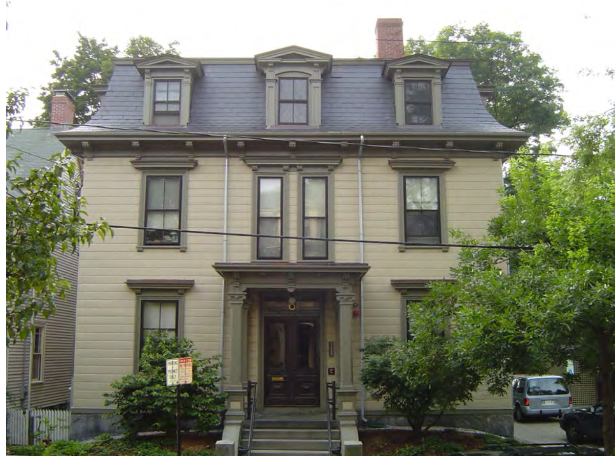
The conversion of a historic building on Bigelow Street into 10 studio and 1-bedroom affordable apartments was approved via a comprehensive permit
