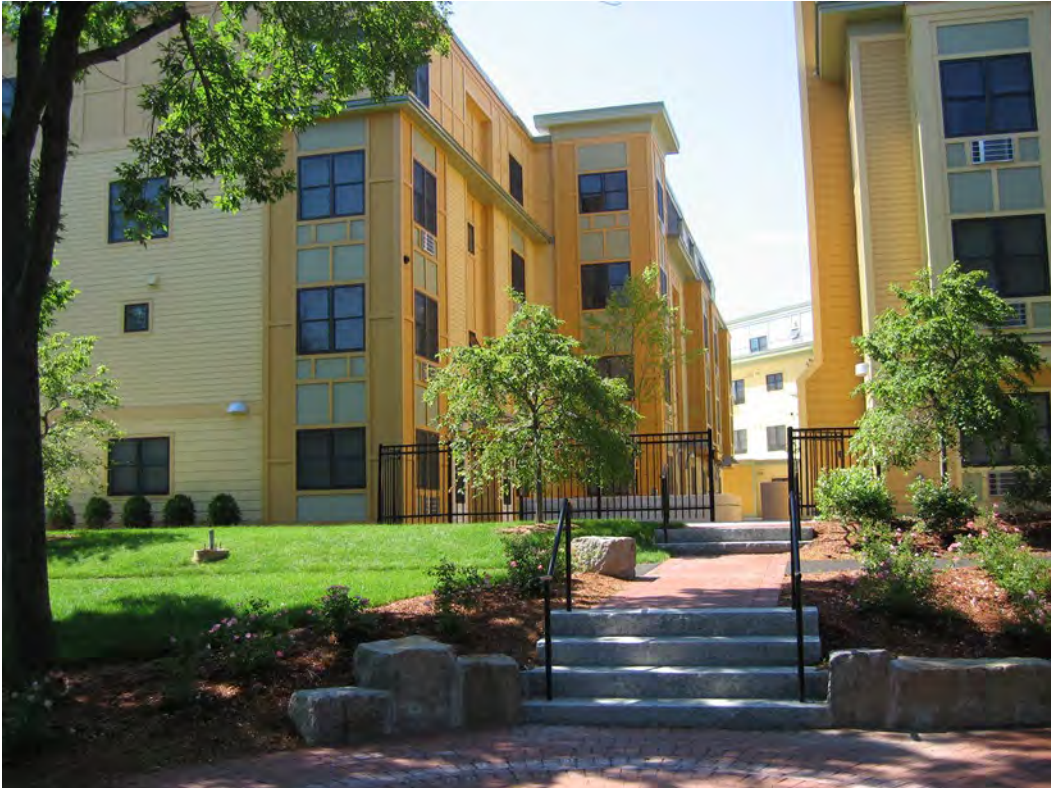
Trolley Square: new construction of 40 affordable units in mixed-use development on former City-owned property; created prior to AHO
