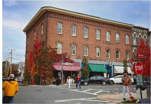
Figure 5. Mixed use commercial and apartments can be a desirable feature within town centers.
